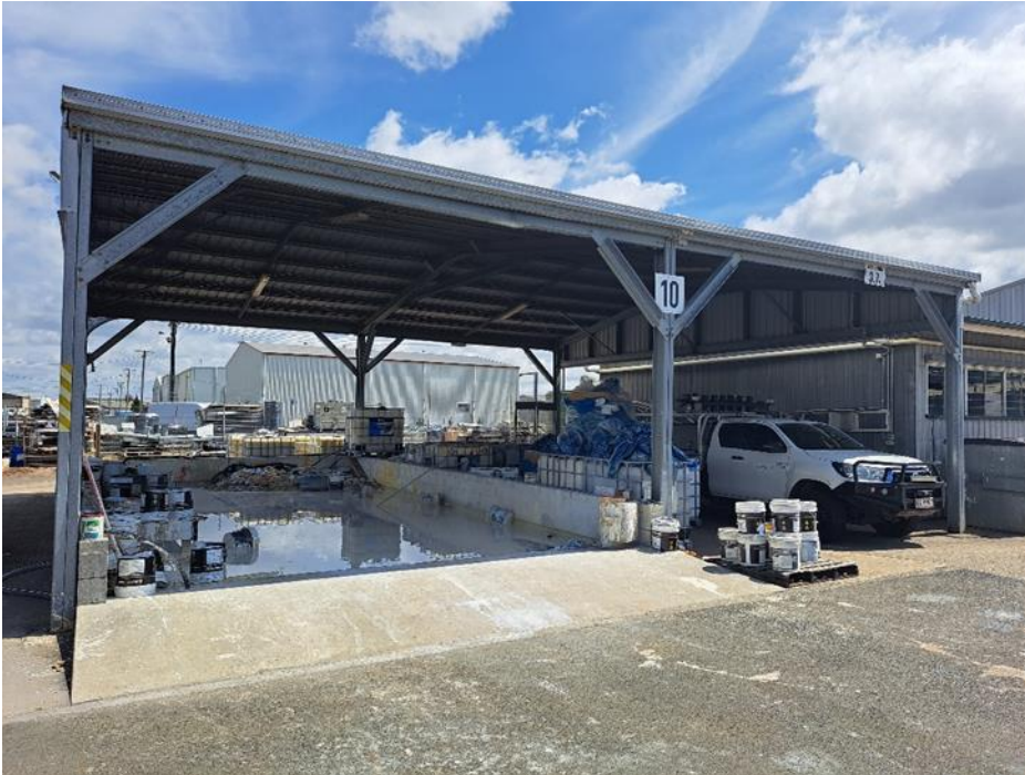
Figure 3.1: Toowoomba linemarking washdown and storage area
