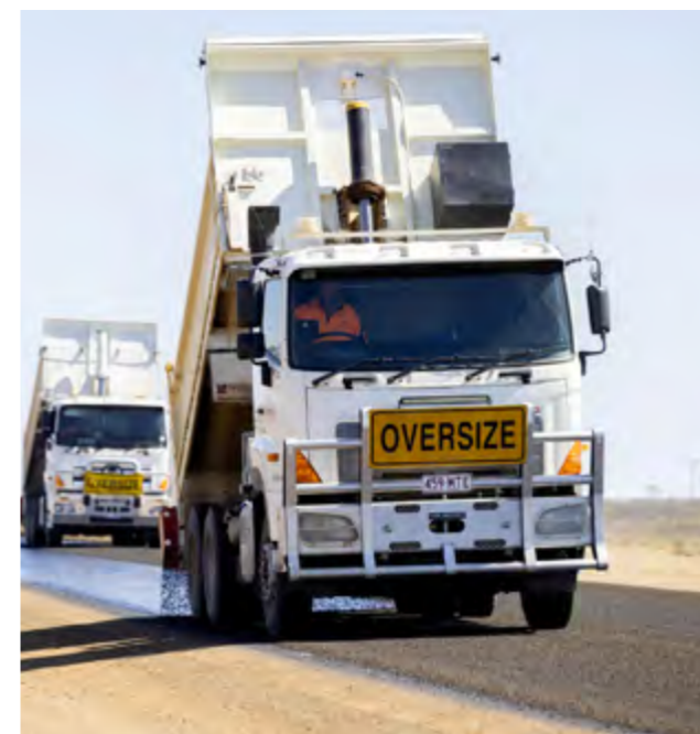
Barcardine- Aramac Road, rehabilitate and widen 2021 Image Source: TMR (2021)
