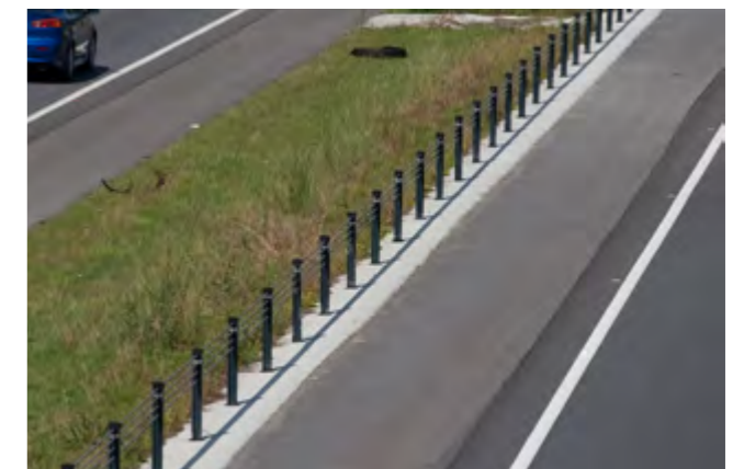
Wire Rope Safety Barrier System on Australian Road. Image Source: NACOE (2021)
