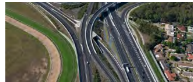
New Deagon Deviation interchange (facing south), Gateway Upgrade North Project, March 2019.
