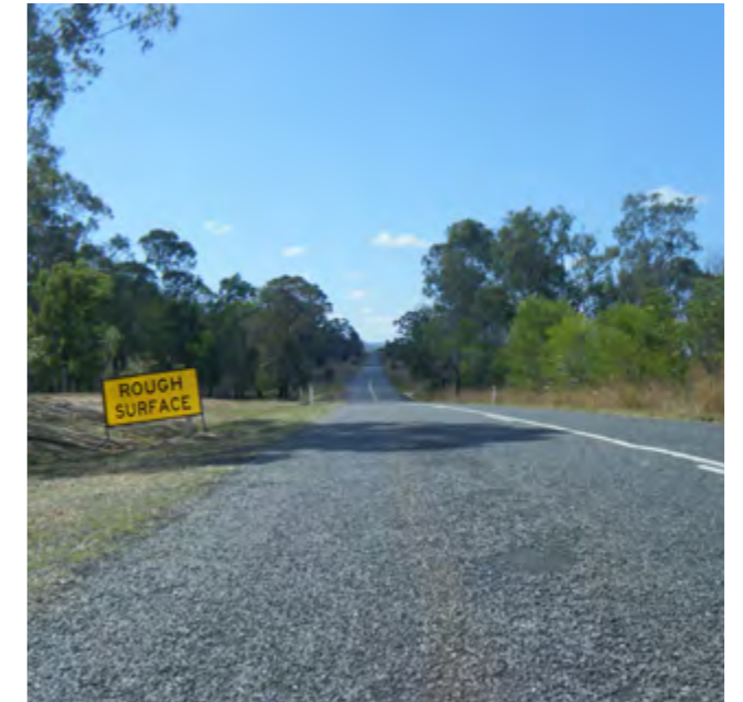
Spray Sealed Road, Rural Queensland Image Source: ARRB (2018)
