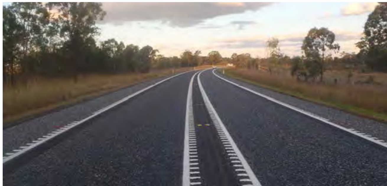
Wide centrelines on the Bruce Highway Image Source: TMR (2015)
