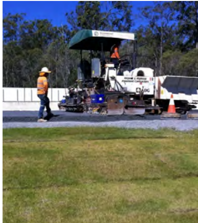
Forming of upper HSG base layer using paver. Image Source: NACOE (2018)
