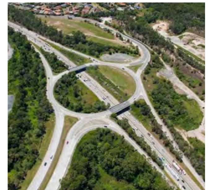
Aerial view of construction works Bicentennial Road interchange Source: TMR (2017)
