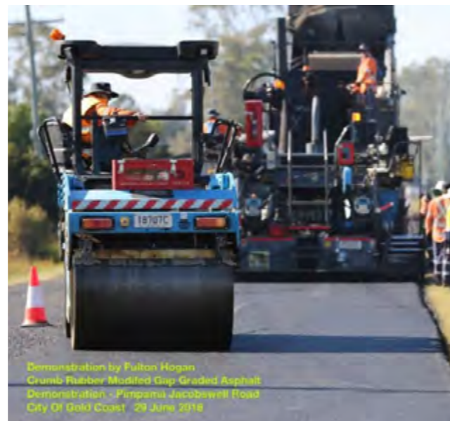
Demonstration by Fulton Hogan, Crumb Rubber Modified Gap Graded Asphalt Demonstration - Pimpama Jacobs Well Road City of Gold Coast.
