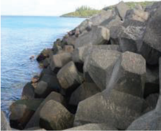
Figure 2.12: Accropode breakwater blocks in situ
