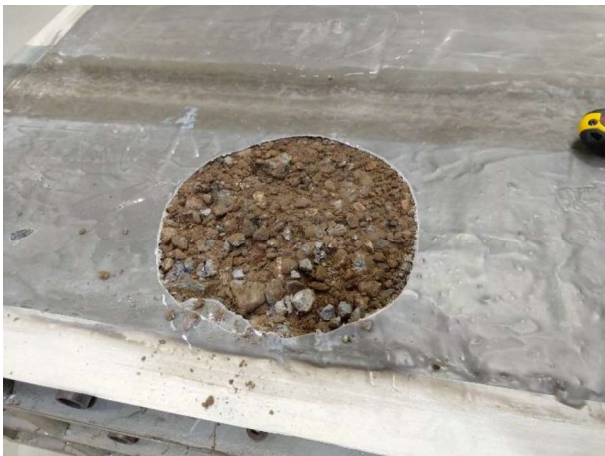
Figure G.17: Preparation for sand replacement
