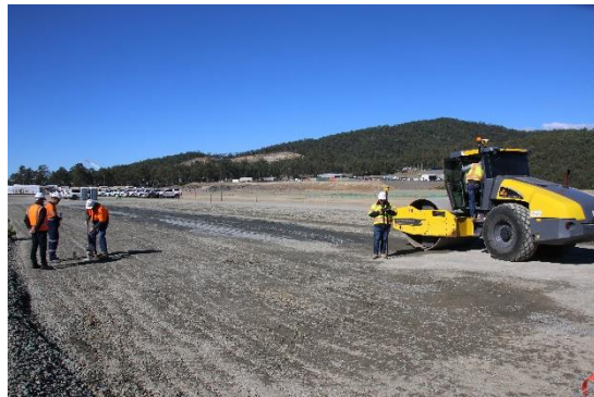
IC Roller and, In-situ Spot Tests
