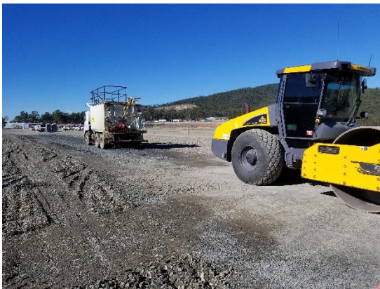
Moisture conditioning and roller compaction
