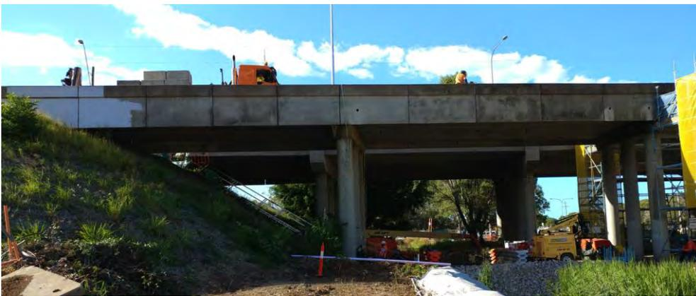
Notes: At the time of the photo, the bridge was undergoing load tests with the RMS truck, which is visible on the deck.
