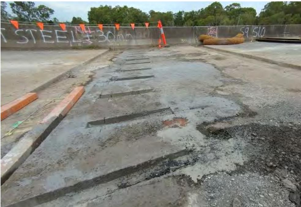
Figure E 7: TSB cuts – View of the bridge deck after cutting of TSB 5 (damaged stage D4B), facing northeast
