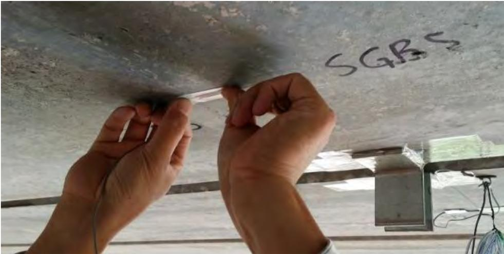
Figure E 2: Instrumentation of the deck soffit – layout
