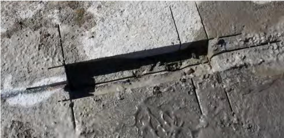
Figure E 6: TSB cuts – View of the bridge deck after cutting of TSB 2 (damaged stage D4A), facing south
