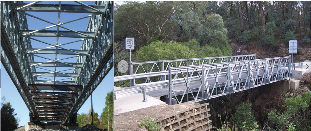
Figure 3.6: C-200 bridge superstructure
