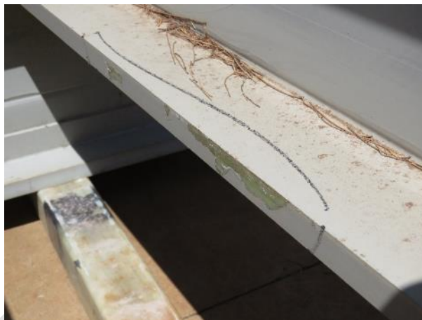
Figure 3.14: Typical defective finishing surfaces noted at the end of girder type S3
