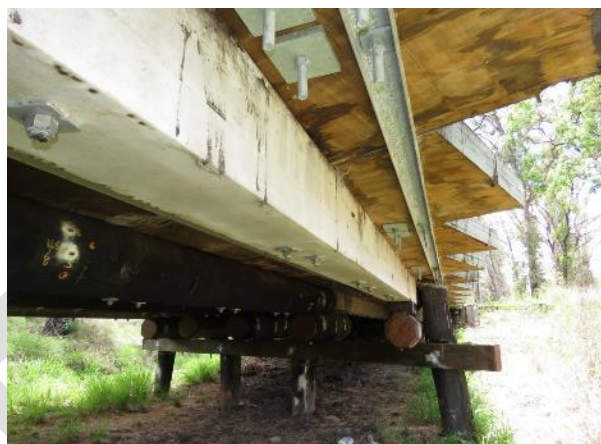
(b) View of FRP girder on Span 2 (S2-G1)
