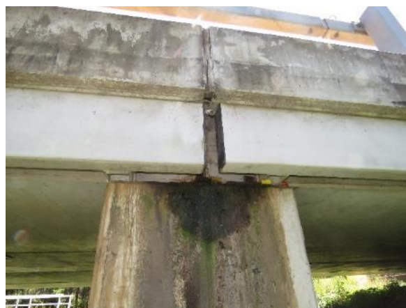
Figure 6.12: Water leak on pier headstock
