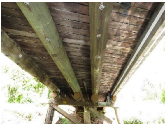
(a) view of the FRP girder from below
