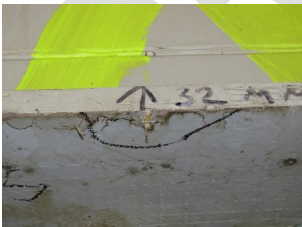
Figure 5.8: Minor chipping of the coating at the soffit on LHS on end 2 of S1-G1
