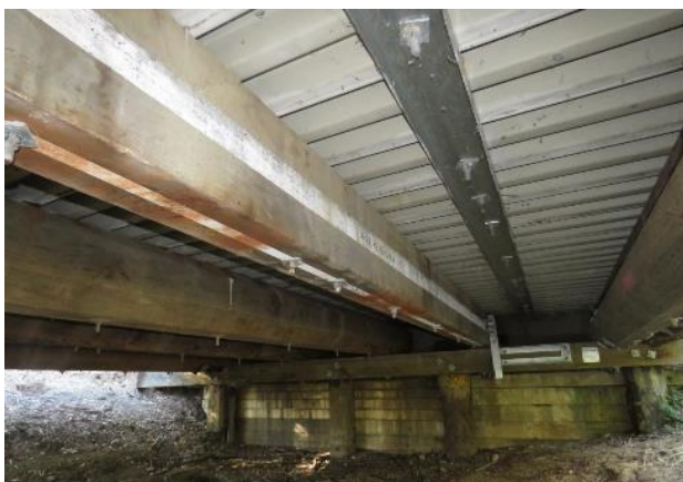
(a) FRP girder on span S1
