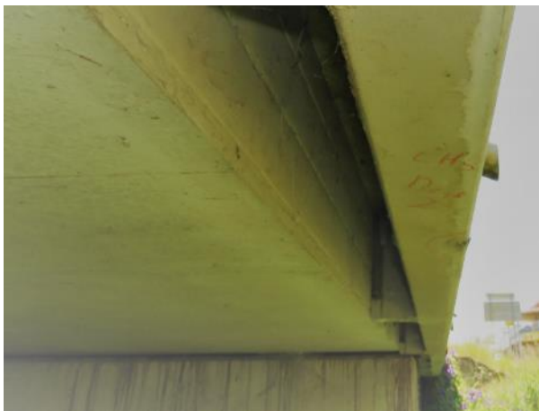
Figure 6.5: Single FRP girder under the kerb
