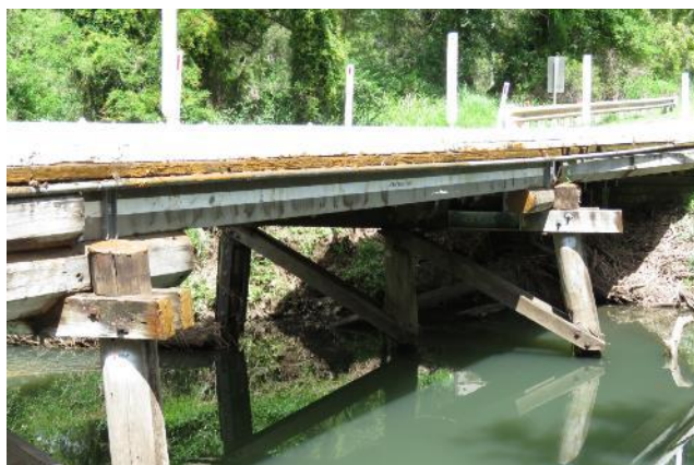
(b) view of the FRP girder from side
