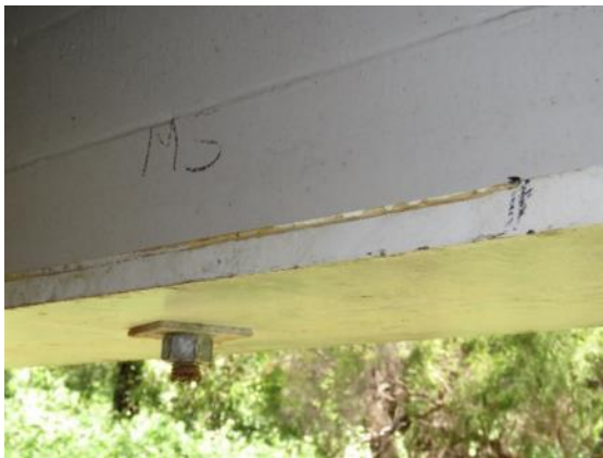
Figure 5.8: Minor chipping of the coating at the soffit on LHS on end 2 of S1-G1
