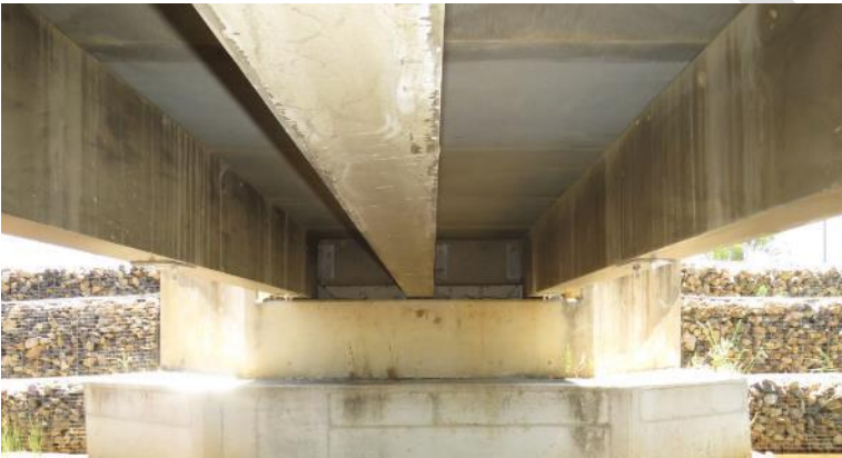
Figure 6.18: No cracking observed at water leak areas on internal faces of girders
