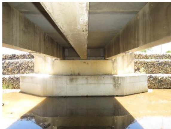
Figure 6.16: View from approach 1
