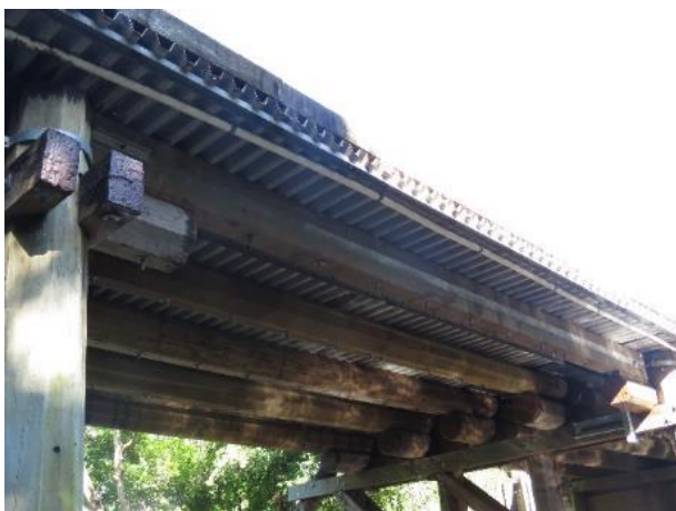
Figure 5.25: View of FRP girder on Obi Ck No1 Bridge (external girder)
