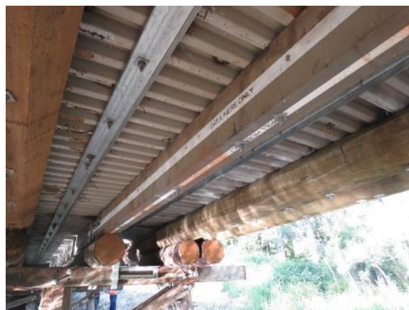
(b) FRP girder on span S3
