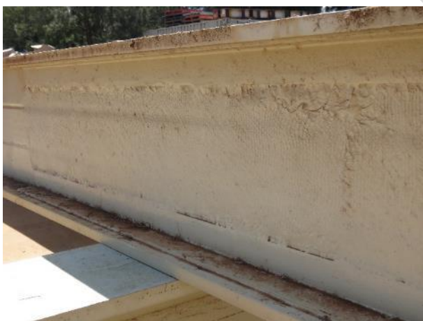
Figure 3.14: Typical defective finishing surfaces noted at the end of girder type S3
