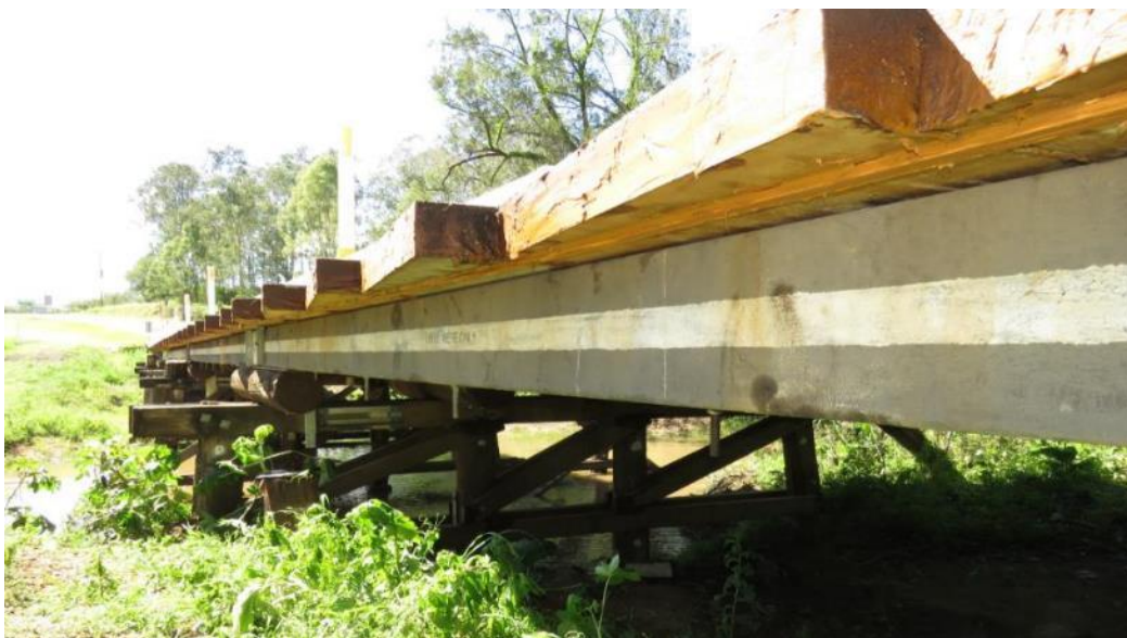
Figure 5.13: Todd Bridge – view of FRP replacement girders
