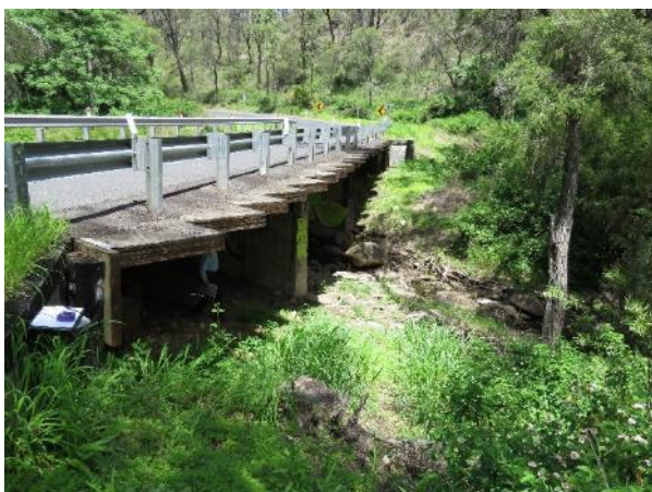
(a) General view of bridge from RHS
