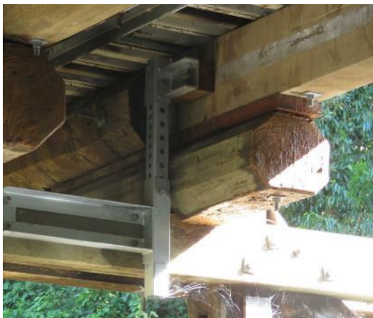
Figure 5.30: Good contact with packers and corbel
