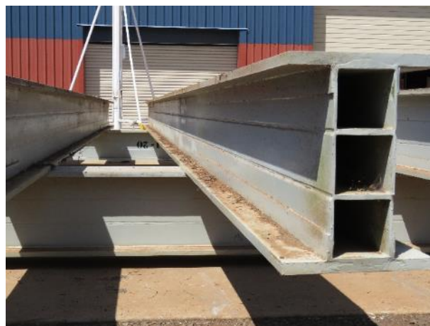
Stockpiled girder type S2
