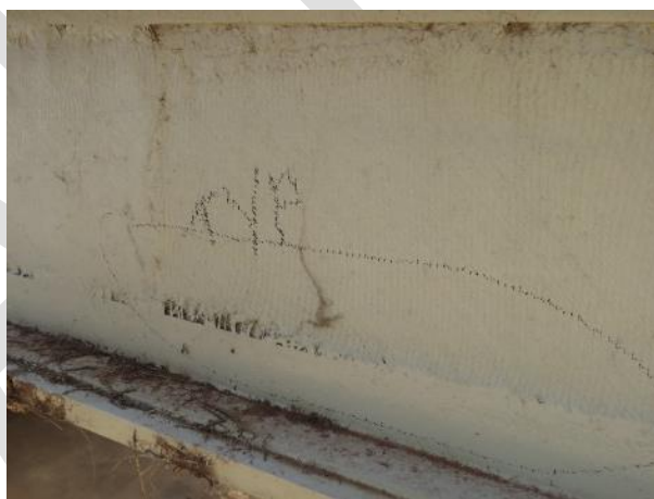
Figure 3.14: Typical defective finishing surfaces noted at the end of girder type S3
