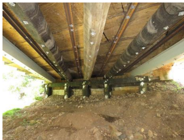
(b) View of FRP girders on Span 1
