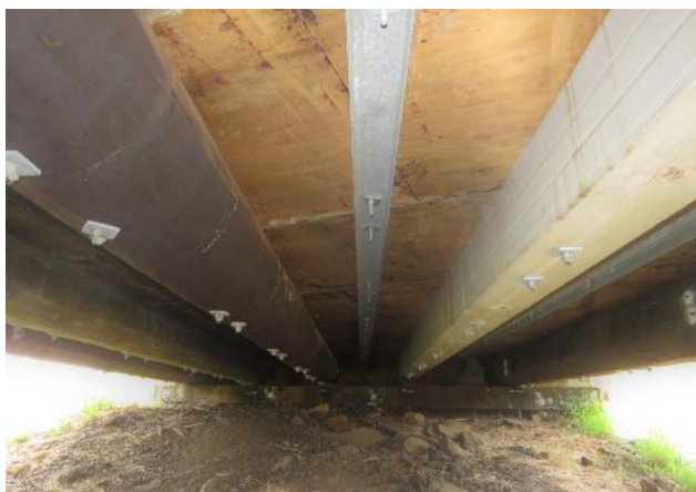
(a) View of FRP girder on Span 1 (S1-G2)
