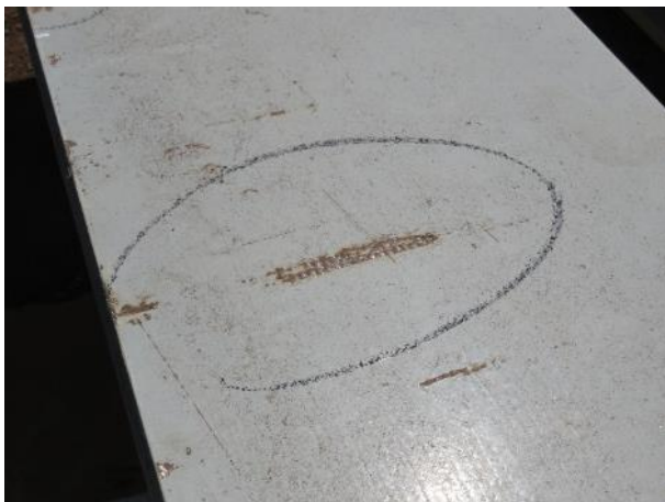
Figure 3.14: Typical defective finishing surfaces noted at the end of girder type S3
