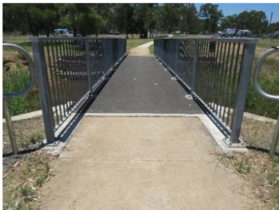
Figure 6.15: Left-hand side view of Sandy Pedestrian Bridge
