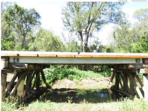
Figure 5.18: WCFT FRP girder on span S5
