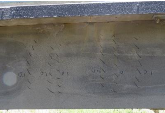
On girder G1
