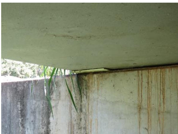
Figure 6.6: FRP sheet used as a packer on the headstock
