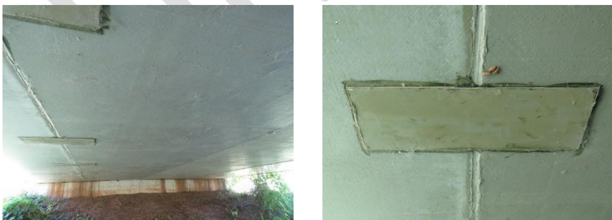
Figure 6.4: Transverse pads at soffit of bridge
