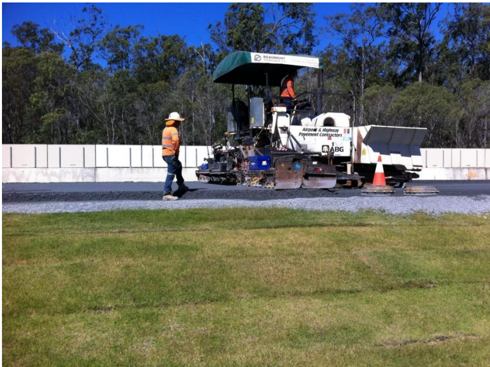
Figure 4.10: Forming of upper HSG base layer using paver
