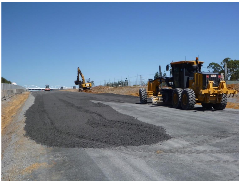
Figure 4.11: Forming of upper HSG base layer using motor grader
