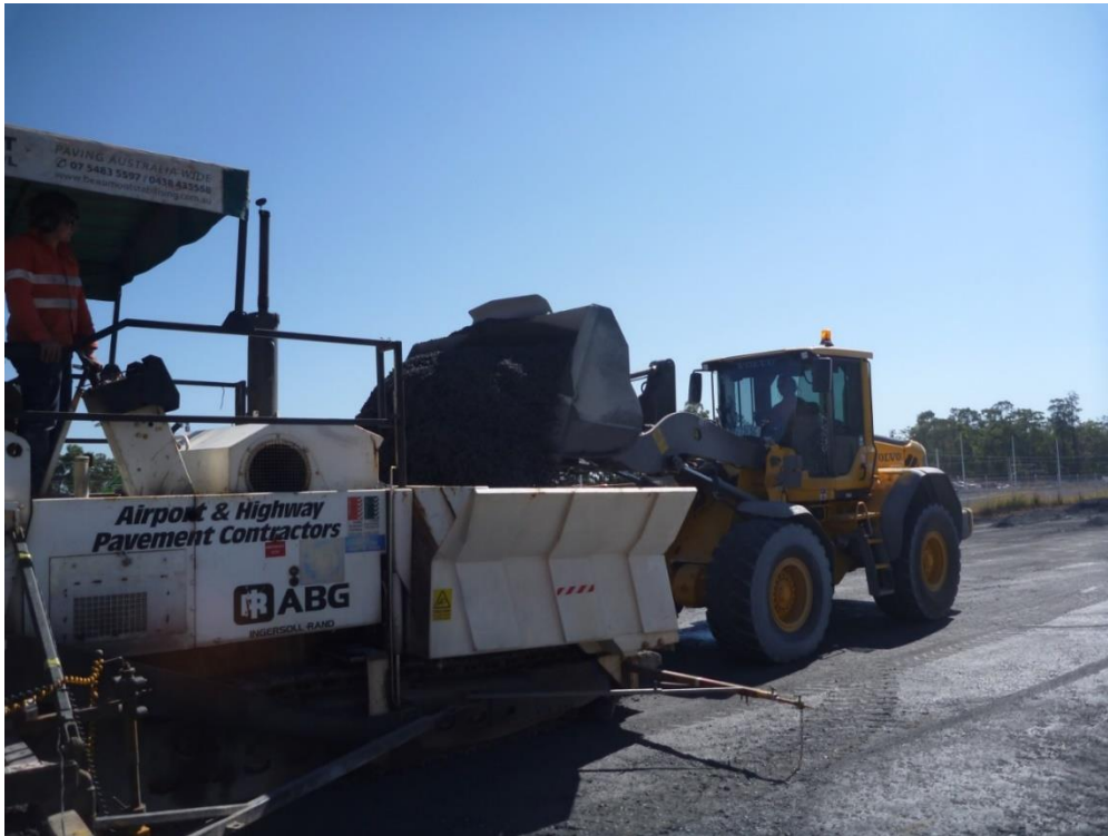
Figure 4.9: Front-end loader filling aggregate hopper of paver
