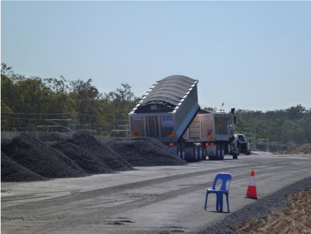
Figure 4.8: HSG base material being delivered and formed into stockpiles
