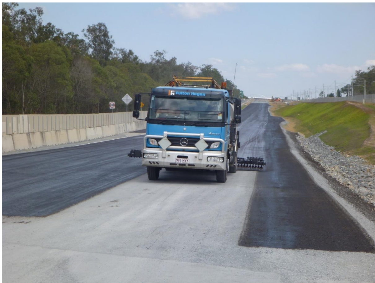
Figure 4.23: Application of prime coat to prepared HSG base
