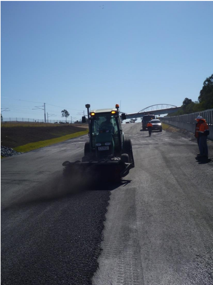
Figure 4.22: Removal of surface debris before application of prime coat
