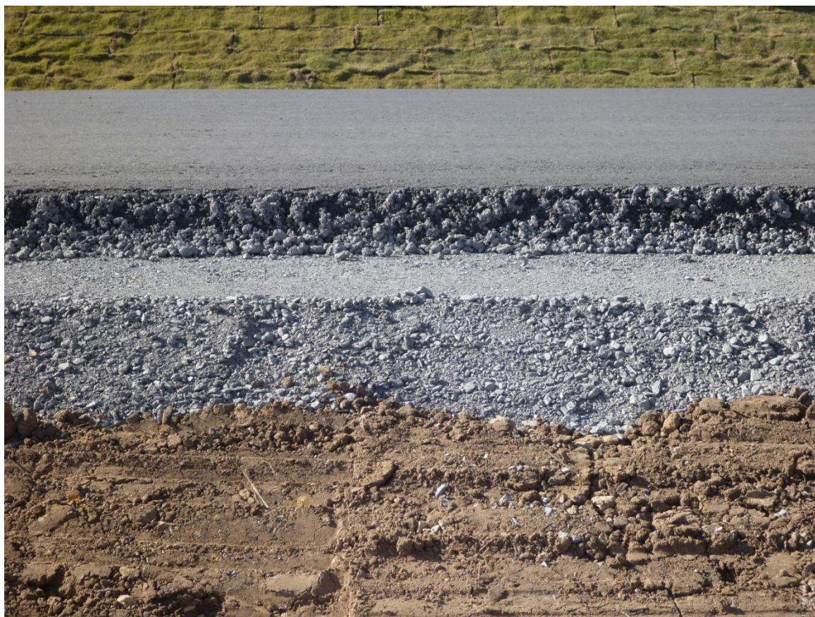
Figure 4.4: Pavement cross-section including lower HSG base, upper subbase, lower subbase and natural subgrade
