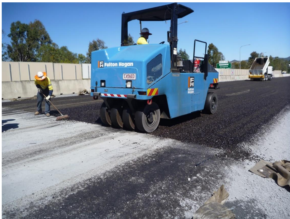
Figure 4.26: Rolling of the 14 mm sealing aggregate
