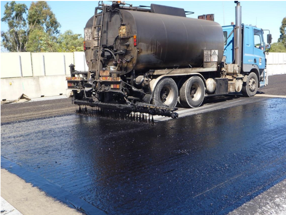
Figure 4.24: Application of initial PMB seal
