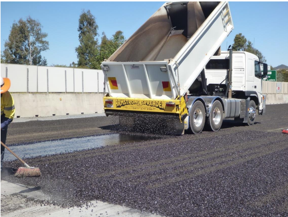
Figure 4.25: Spreading of 14 mm sealing aggregate
