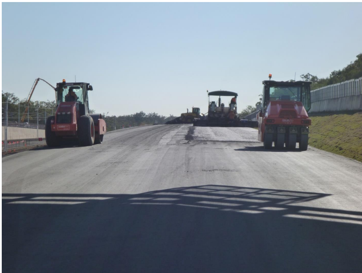
Figure 4.12: Compaction equipment used on the project, including vibrating smooth drum (left) and pneumatic tyred (right) rollers
