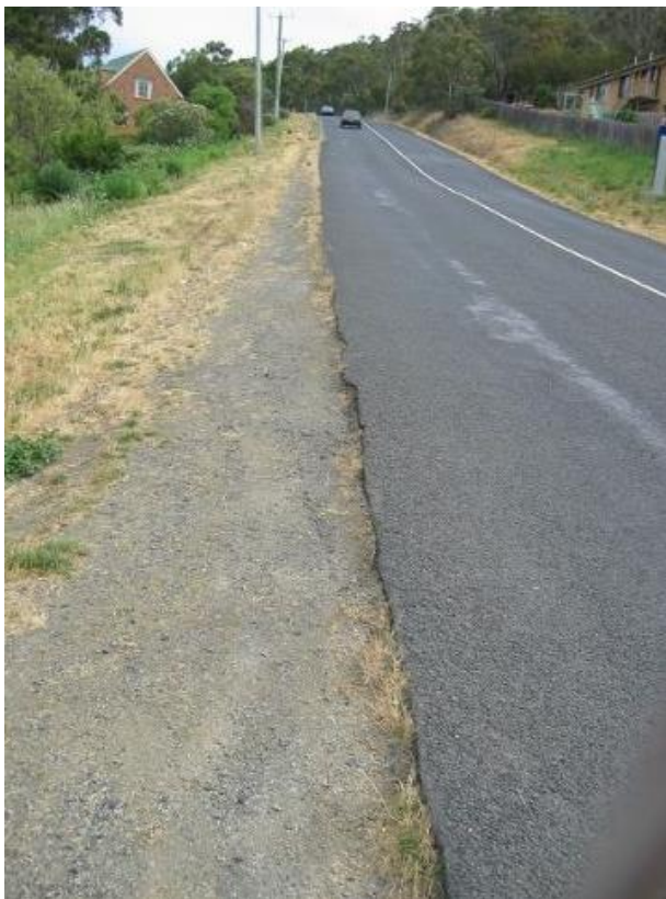
Figure 5.24: Edge drop along shoulder
