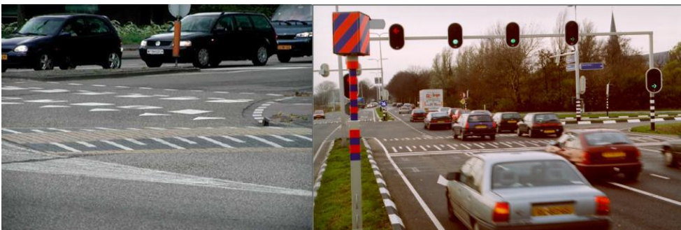
Figure 7.23: Images of speed humps on European Roads (raised stop line or platform)
