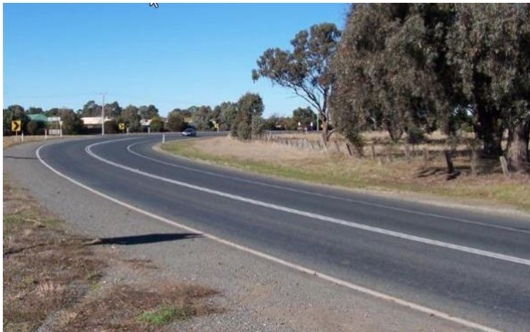
Figure 5.19: Curve widening on shoulders
