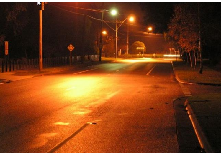
Figure 7.3: Street lighting on approach to roundabout
