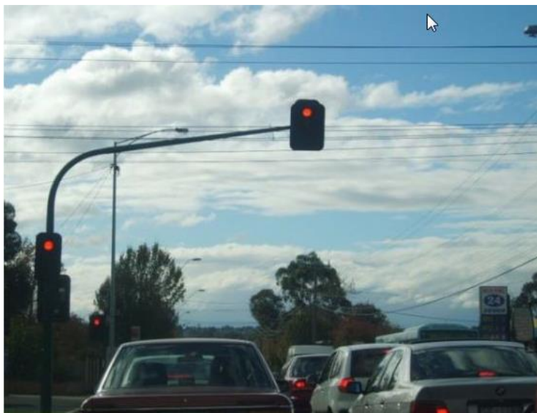
Figure 7.4: Traffic signal displays mounted on a mast arm
