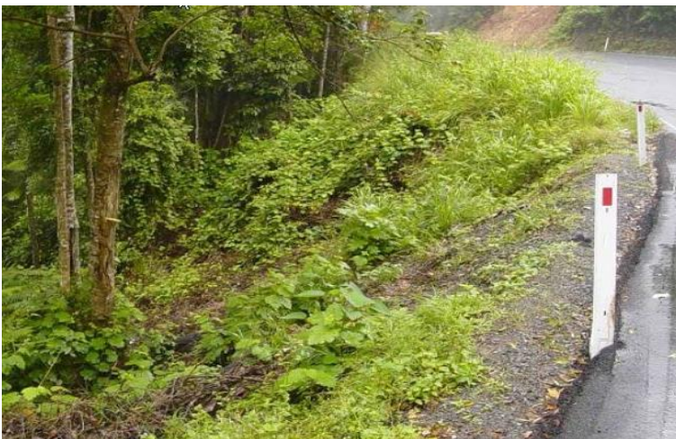
Figure 6.5: Steep embankment within the clear zone
