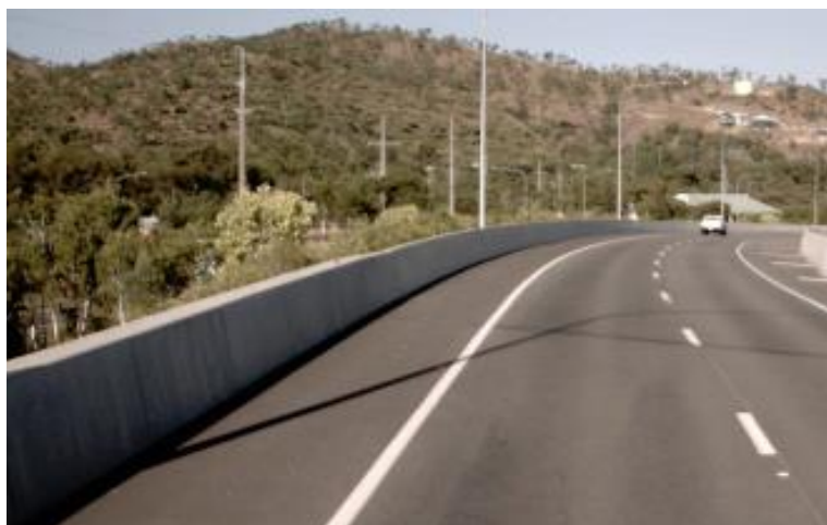
Figure 6.6: Rigid concrete safety barrier
