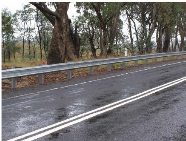
Figure 6.7: Semi rigid W-Beam safety barrier
