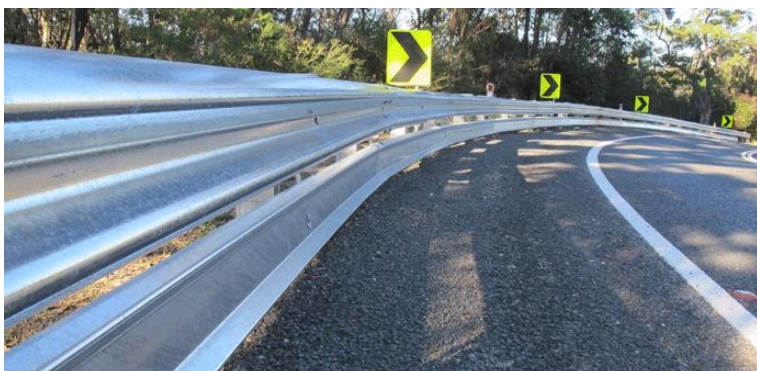
Figure 6.11: Under-run protection for motorcyclists on W-Beam safety barrier
