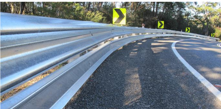
Figure 5.7: Under-run protection for motorcyclists on W-Beam safety barrier
