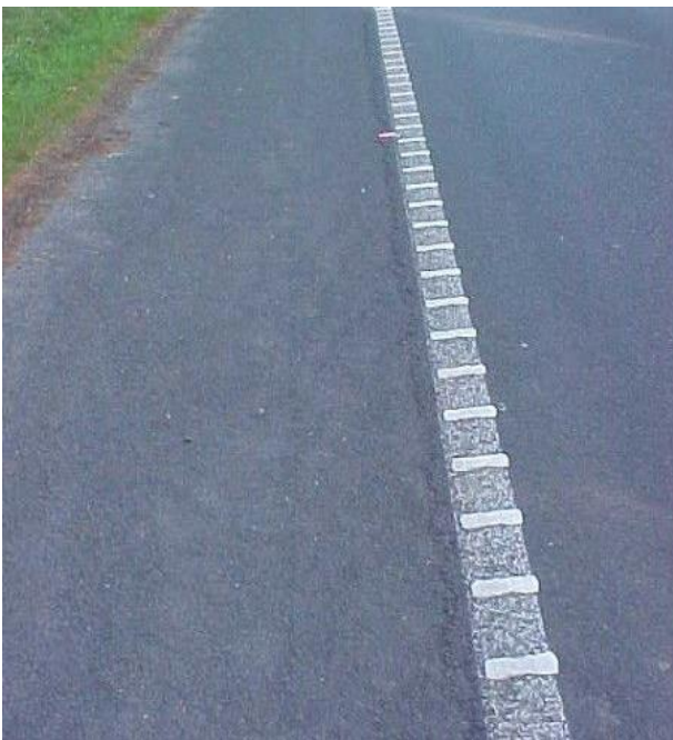
Figure 6.2: A longitudinal rumble strip or raised profile edge line
