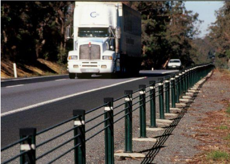
Figure 6.8: Flexible wire rope safety barrier
