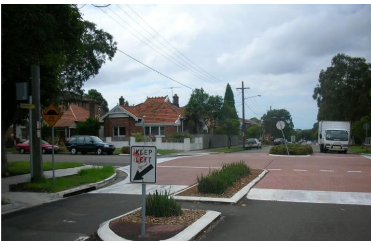
Figure 7.24: Example of an intersection that has been raised and paved a different colour
