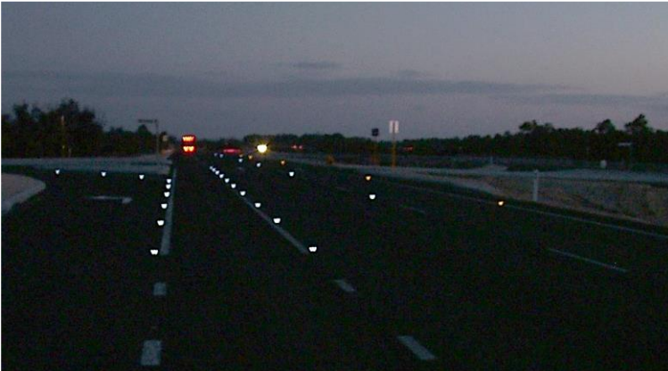
Figure 5.10: Example of internally-illuminated pavement markers at night
