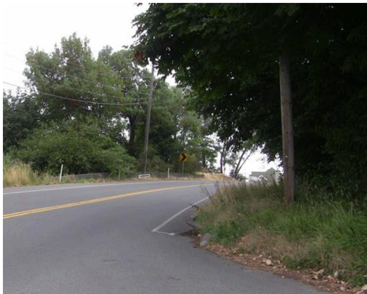
Figure 7.17: Sight distance limited due to intersection being on inside of curve and by vegetation
