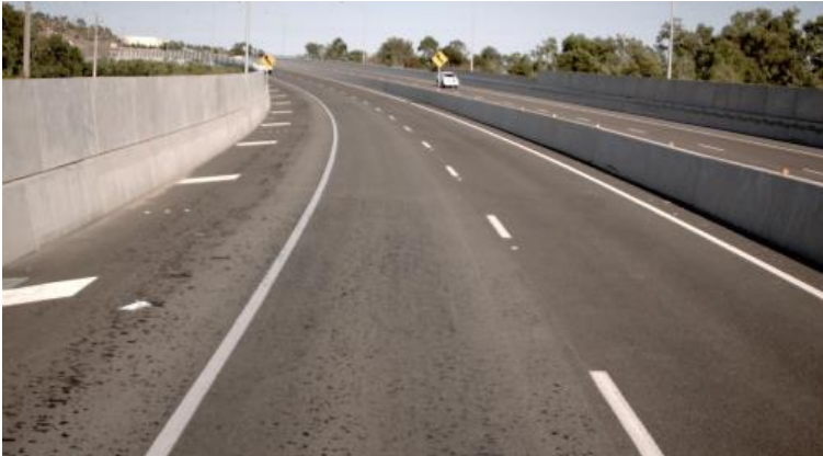
Figure 5.2: Example of a rigid concrete safety barrier
