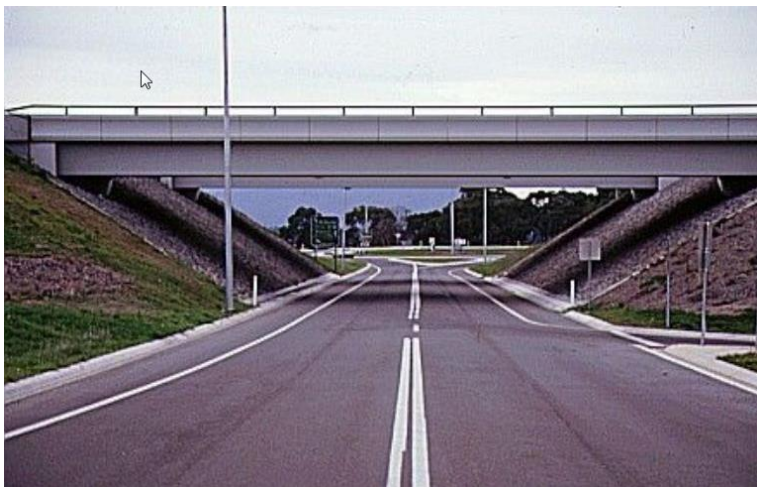
Figure 7.1: Grade separated intersection
