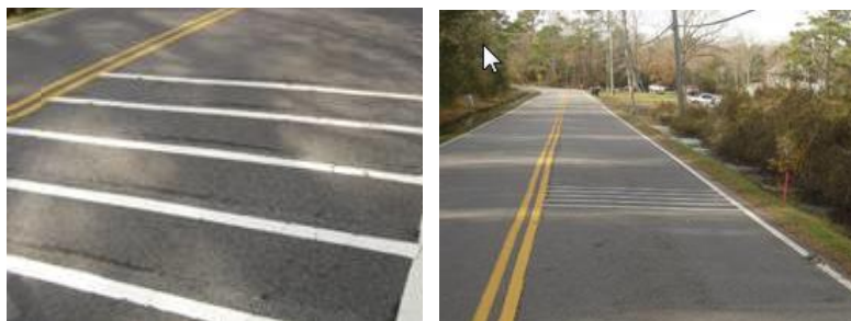
Figure 5.22: Use of transverse rumble strip on approach to curve
