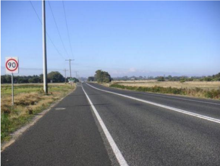
Figure 6.1: Recently sealed shoulder on two lane road
