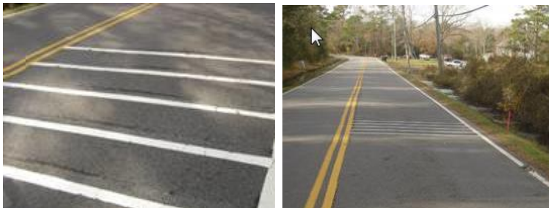
Figure 6.16: Use of transverse rumble strip on approach to curve
