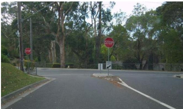
Figure 7.16: Stop signs at a T-junction
