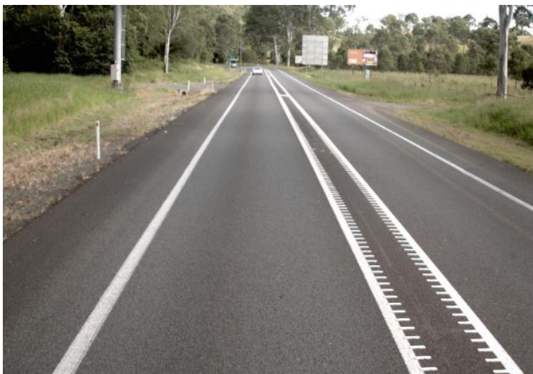
Figure 5.13: Wide centreline treatment with raised profile line-marking on Bruce Highway
