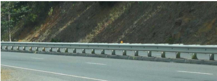
Figure 5.3: Example of a semi rigid W-Beam safety barrier
