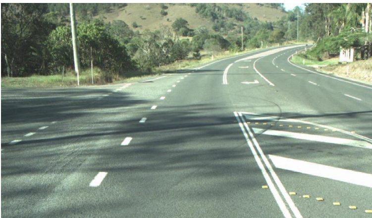
Figure 7.7: Right turn lane in rural area
