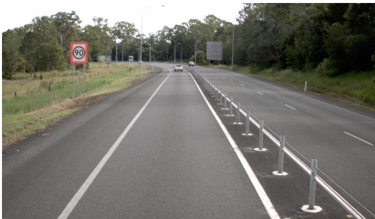
Figure 5.18: Typical 2+1 road configuration
