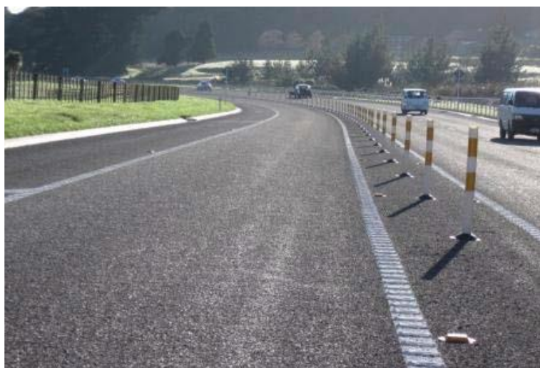
Figure 5.16: Safe-hit posts in central median New Zealand
