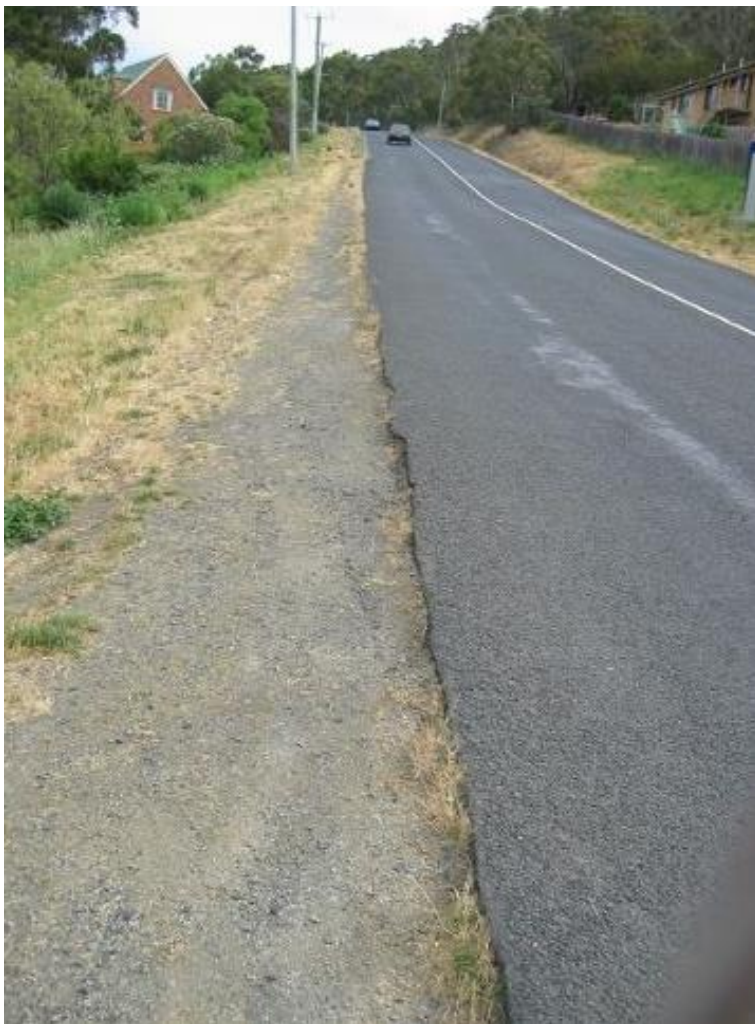
Figure 6.19: Edge drop along shoulder
