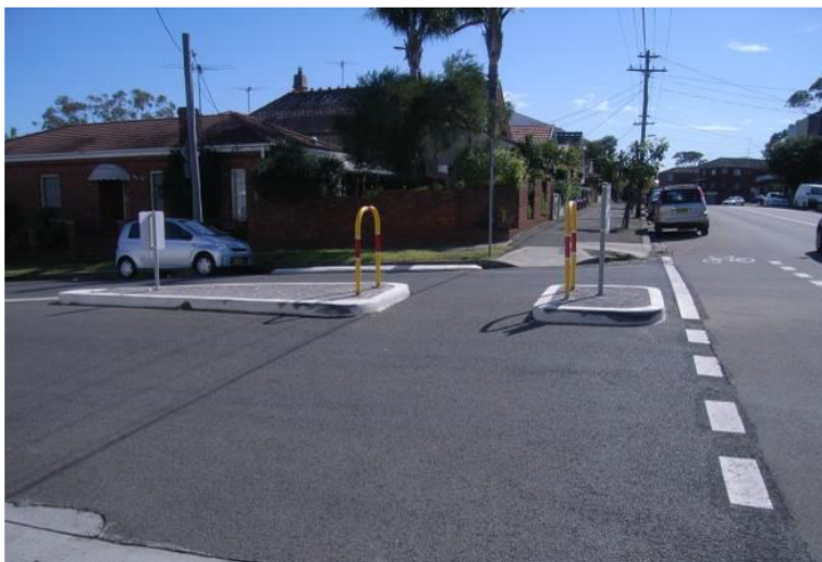
Figure 7.8: Splitter island with a pedestrian refuge
