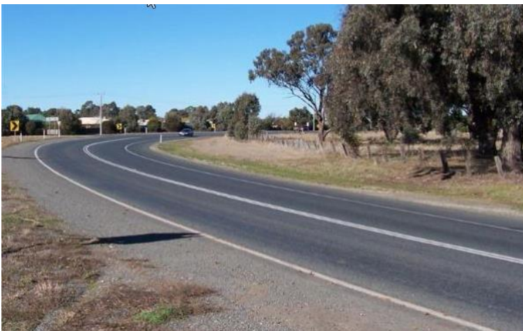
Figure 6.13: Curve widening on shoulders
