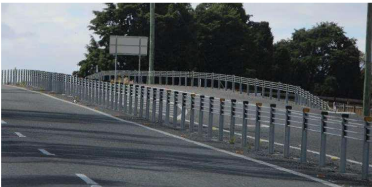
Figure 5.4: Example of a flexible wire rope safety barrier
