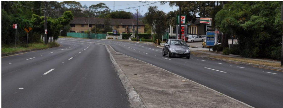
Figure 5.14: Example of a paved raised median
