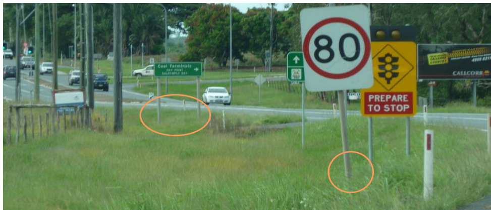
Figure 7.25: Example of roadside hazards at intersection
