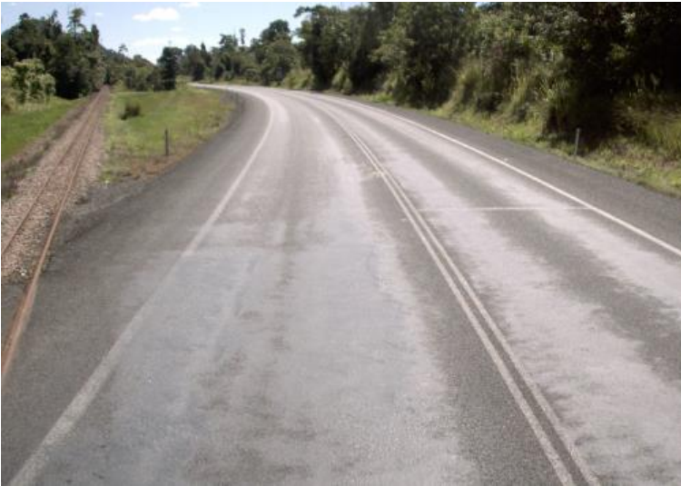
Figure 6.18: Poor skid resistance – polished road surface
