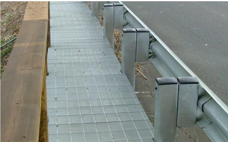
Figure 5.6: Guardrail post caps
