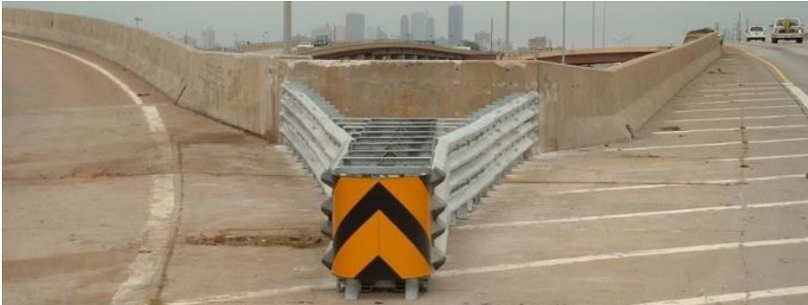
Figure 6.12: Example of a crash attenuation cushion
