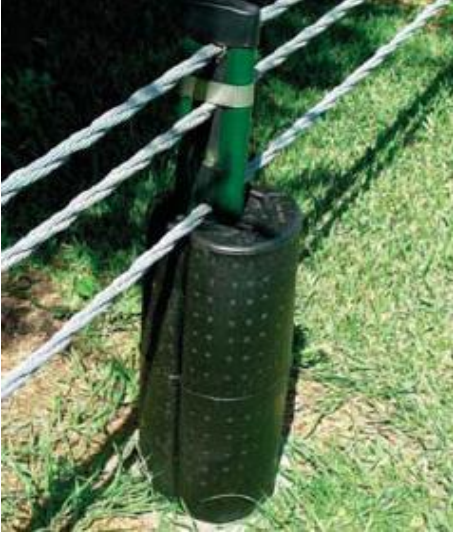
Figure 5.5: Wire-rope barrier post impact absorbing pads
