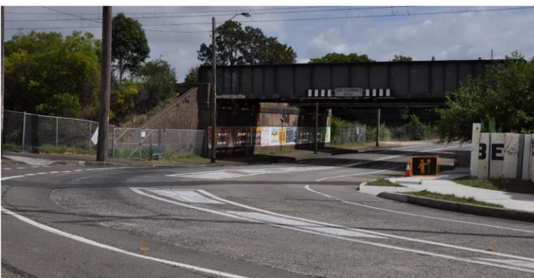
Figure 5.11: Example of a painted median on a curved section of road
