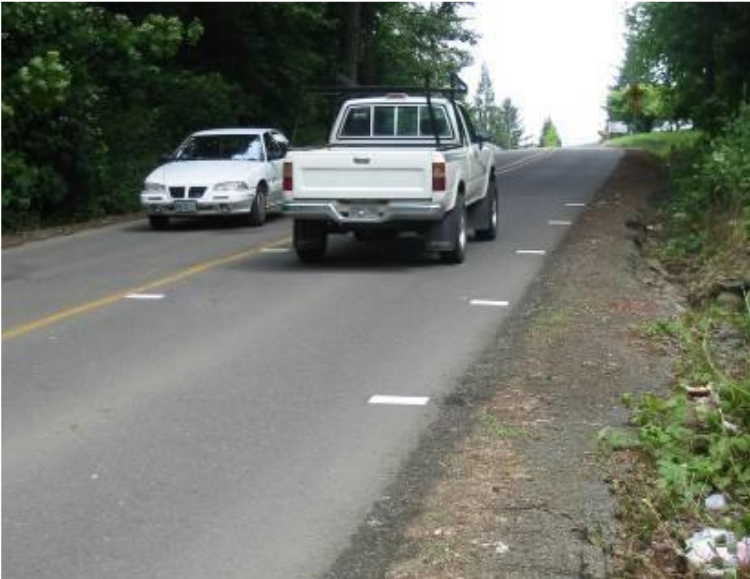
Figure 7.19: Peripheral bars on approach to intersection
