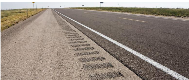
Figure 6.3: Milled rumble strips adjacent to edgeline
