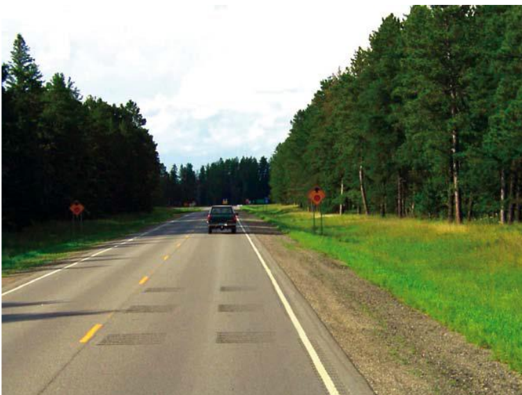
Figure 7.21: Transverse rumble strip on approach to stop-controlled intersection
