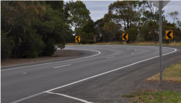
Figure 5.20: Delineation of curve using CAMS
