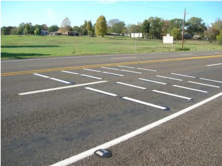
Figure 7.20: Transverse rumble strips
