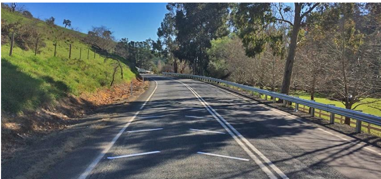
Figure 7.18: Transverse linemarking on approach to rural intersection
