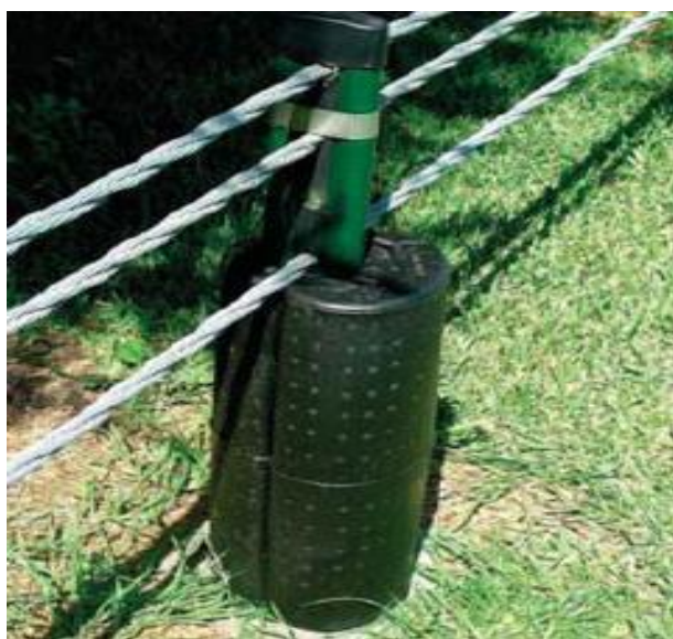
Figure 6.9: Wire-rope barrier post impact absorbing pads
