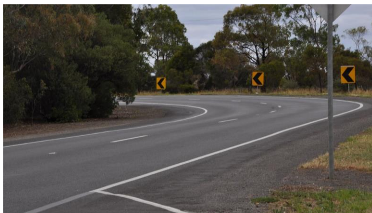
Figure 6.14: Delineation of curve using CAMS
