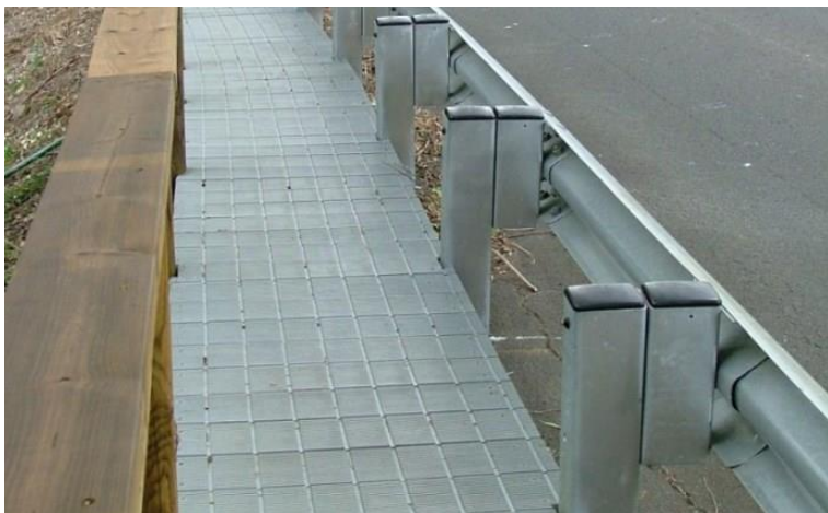
Figure 6.10: Guardrail post caps
