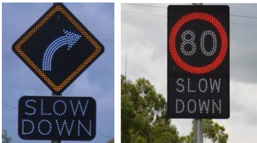
Figure 6.15: Examples of VAS used on approach to curve
