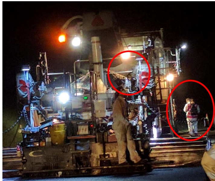
Figure 2. Personal monitoring for particulate matter (PM) during pavement work (red circle)
