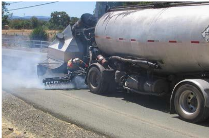
Figure 8.2: Sealing truck with extraction device at spray bar
