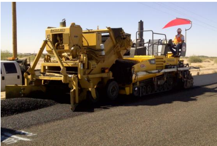
Figure 1.1: Crumb rubber modified asphalt paving operation in California
