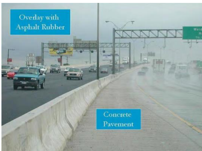
Figure 4.1: Thin porous asphalt used to reduce spray on a concrete freeway in Texas
