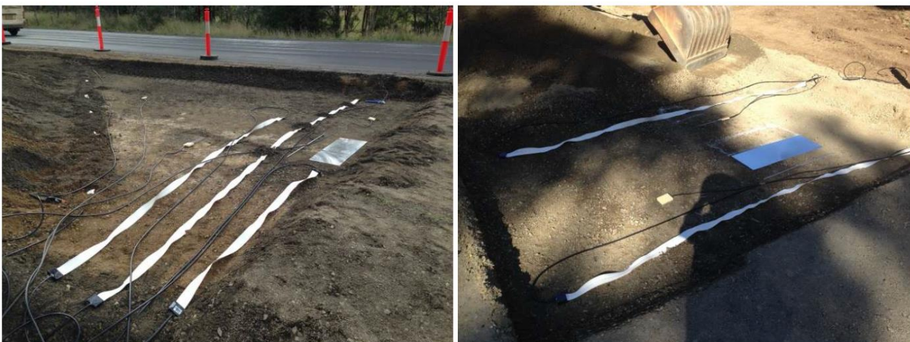
Figure 3.3: 'Ribbon' style TDR sensors and plates at the Cunningham Highway site
