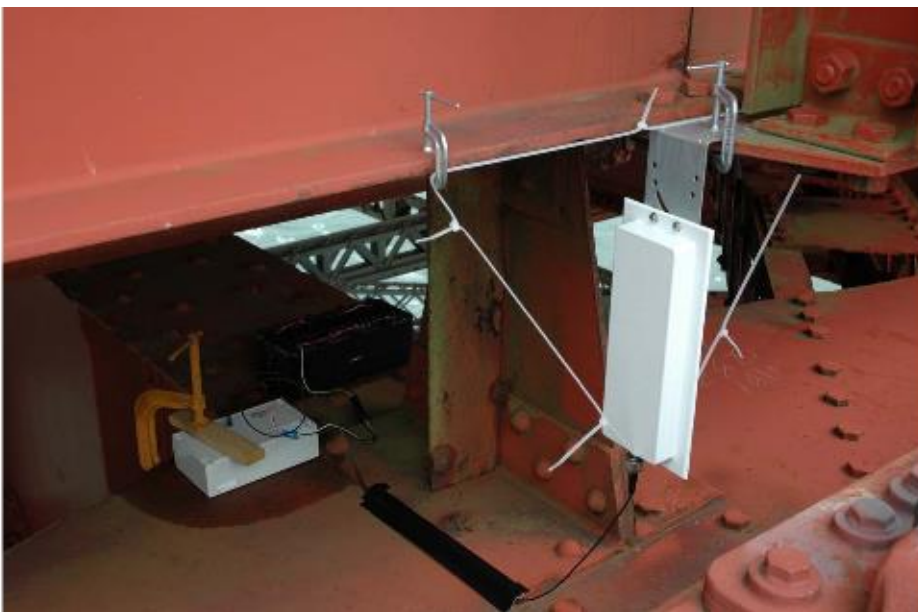
Figure 2.7: The board attached and carefully secured along the main span
