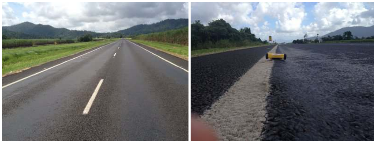
Figure 7.8: Bruce Highway (10N) overview (left) and surface condition (right)
