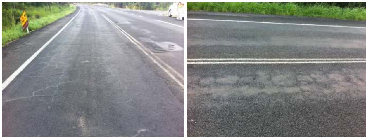
Figure 7.9: Bruce Highway (10N) overview (left) and surface condition (right)
