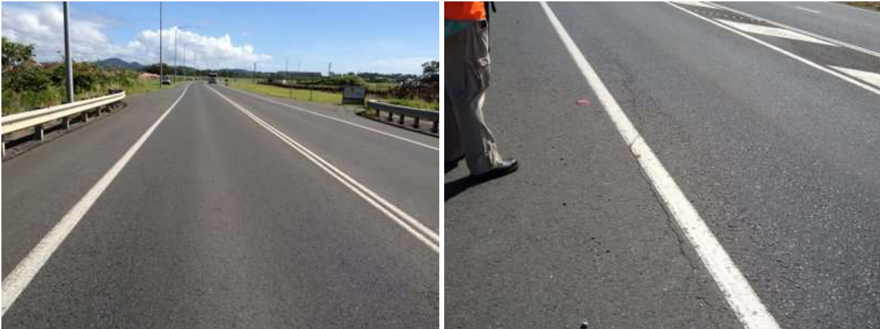
Figure 7.13: Mackay Bypass Road overview (left) and surface condition (right)
