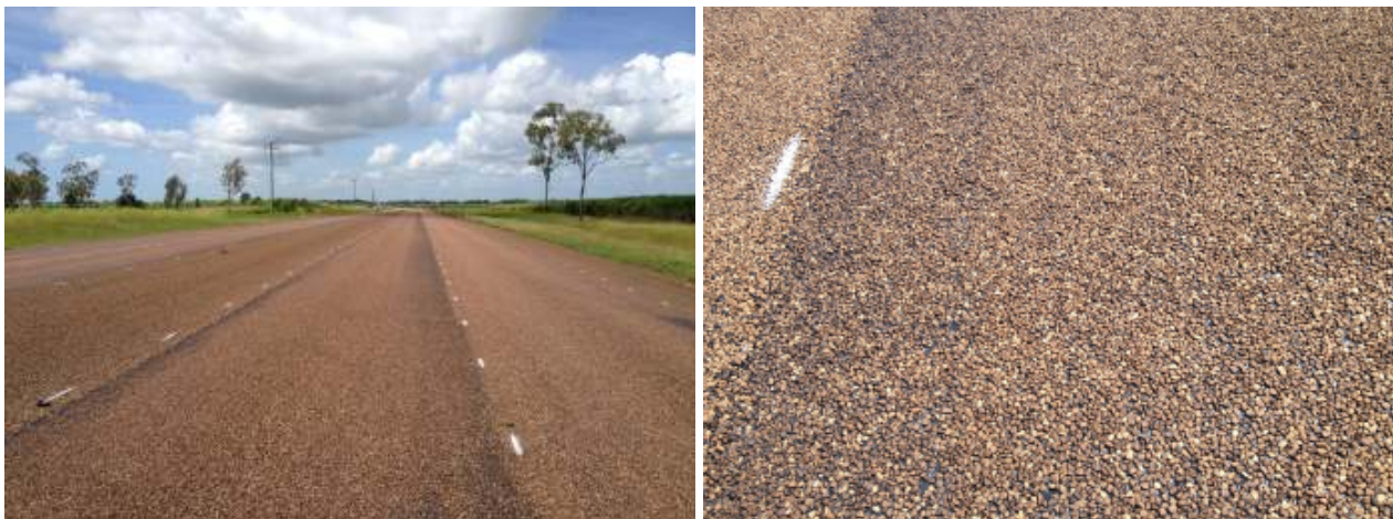
Figure 7.12: Bruce Highway (10L) overview (left) and surface condition (right)
