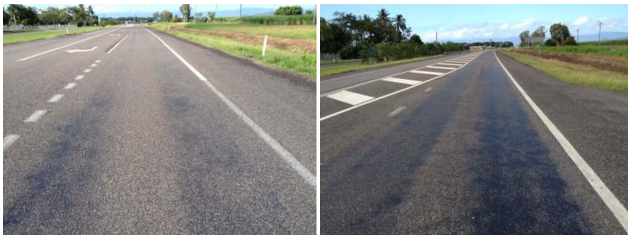
Figure 7.11: Bruce Highway (10M) overview (left and right)
