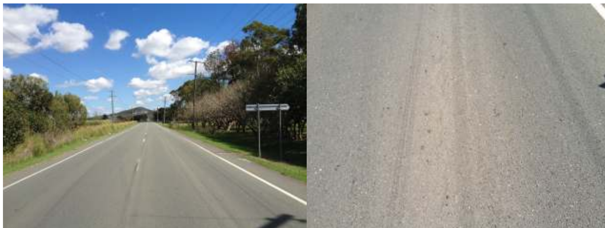
Figure 7.1: Stapylton-Jacobs Well Road overview (left) and surface condition (right)
