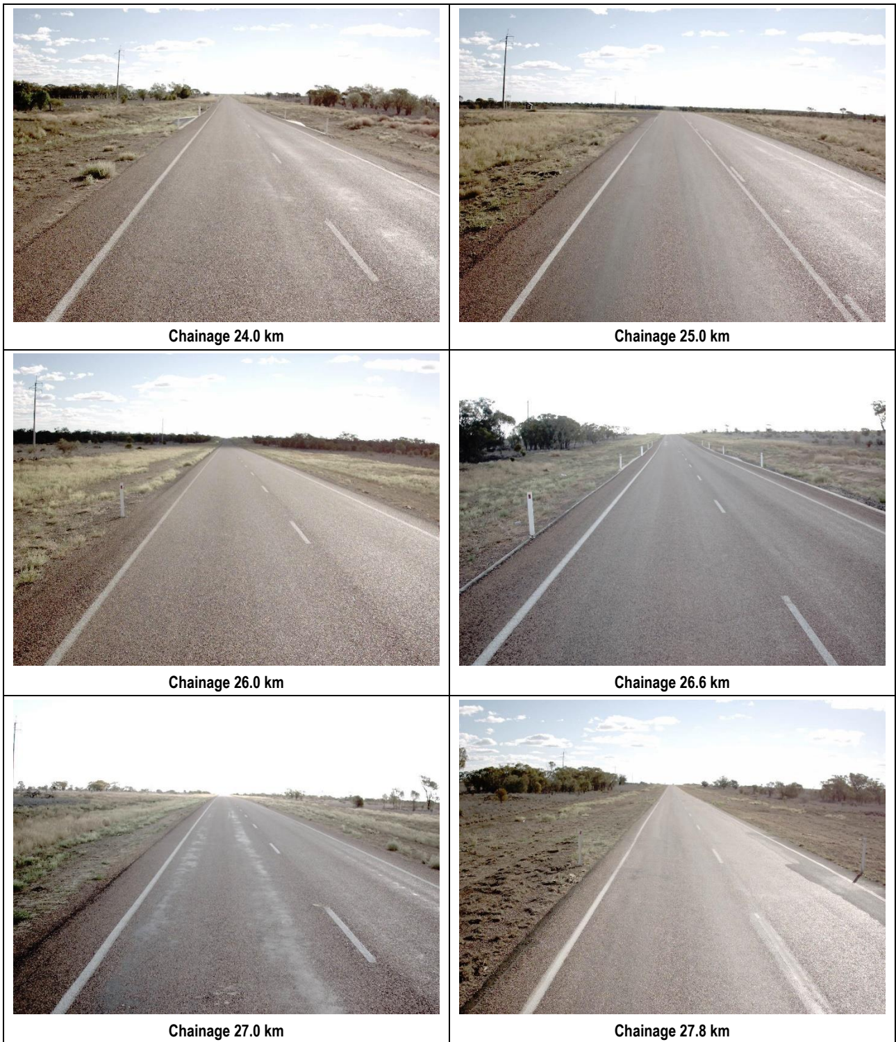
Figure A 3: Visual condition of the monitoring site along Landsborough Highway, 13E
