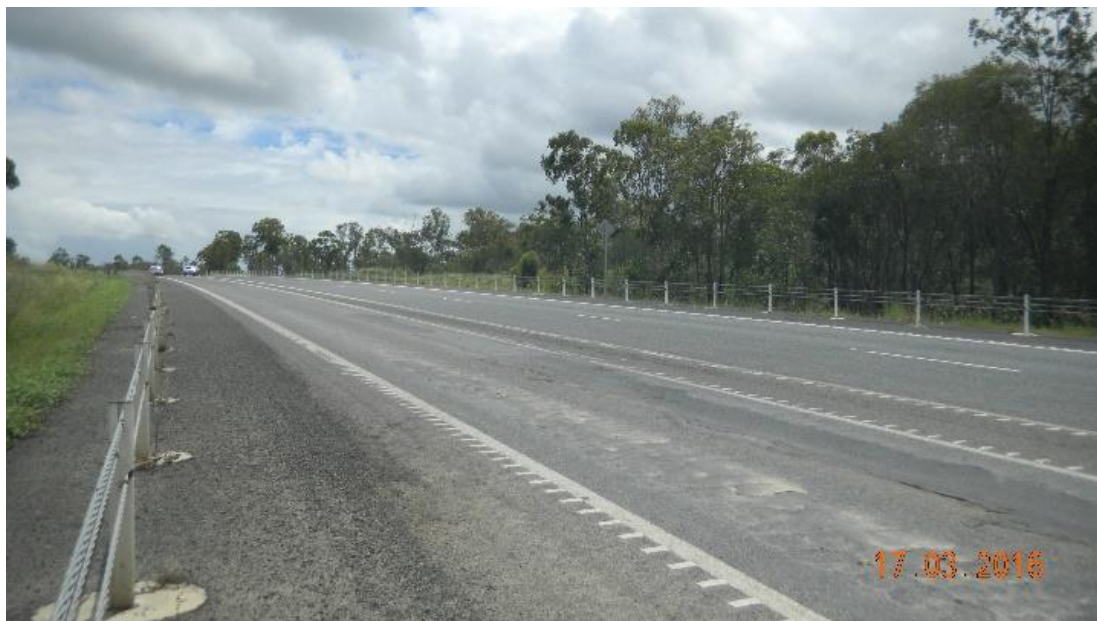
Figure 3.2: Pavement defects observed along Bruce Highway (10D)
