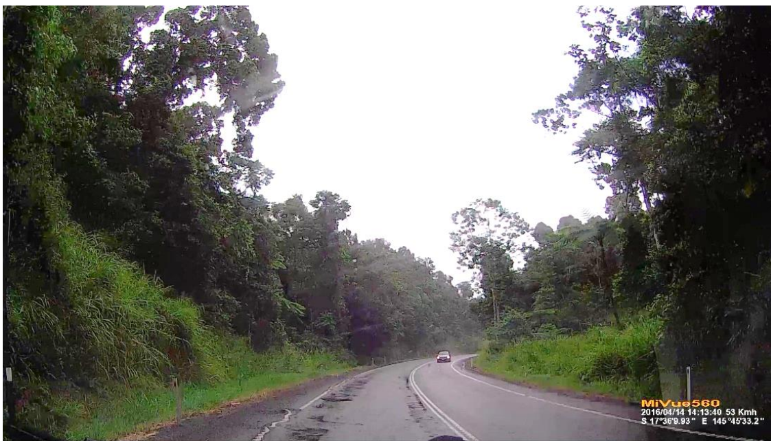
Figure 4.5: Pavement defects observed along Palmerston Highway, 21A, Ch. 29.98–33.92 km
