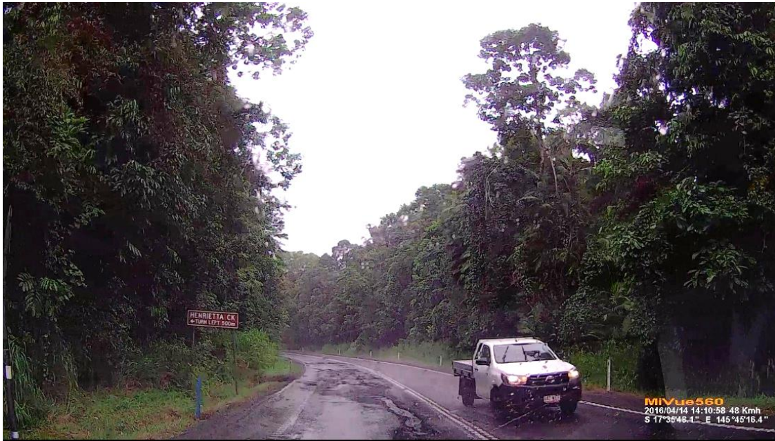
Figure 4.4: Pavement defects observed along Palmerston Highway, 21A, Ch. 29.98–33.92 km
