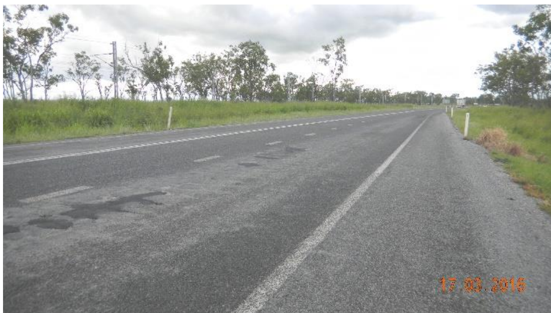
Figure 3.3: Pavement defects observed along Bruce Highway (10E)
