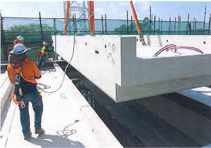
Figure 3.5: Placement of the geopolymer concrete suspended precast panels at the new Global Change Institute building
