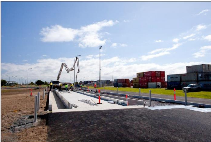
Figure 3.7: Placement of the geopolymer concrete pavement for a weighbridge at Port of Brisbane
