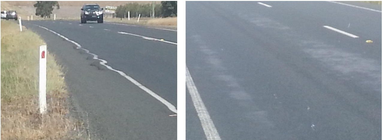
Figure C 4: Shoving causing edge line distortion and some flushing in the wheel paths
