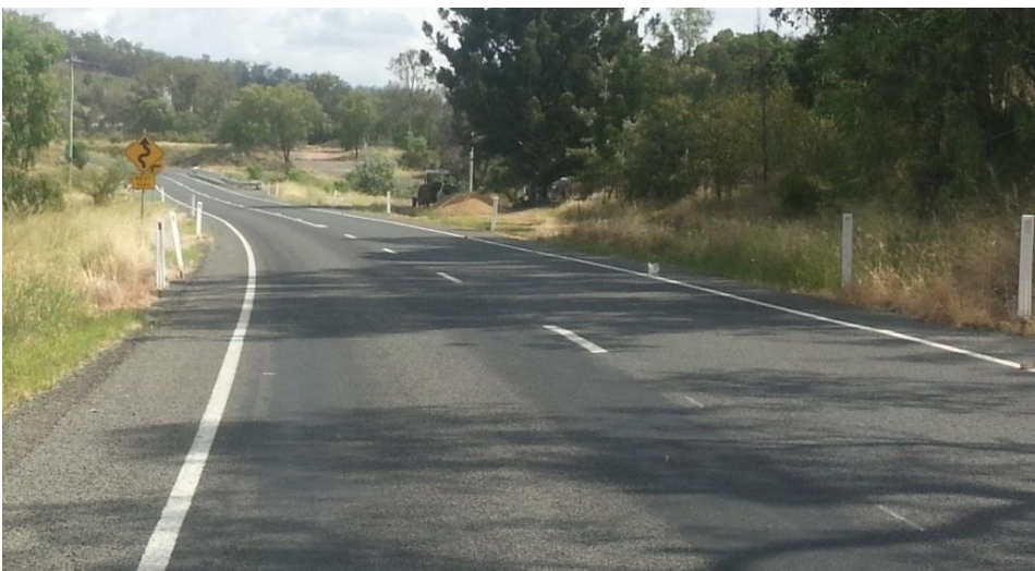
Figure C 5: Minor flushing in the wheel paths
