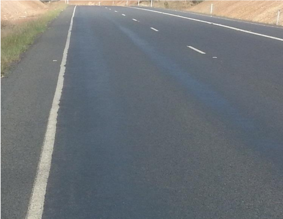
Figure C 3: Some edge line distortion and minor flushing in wheel paths
