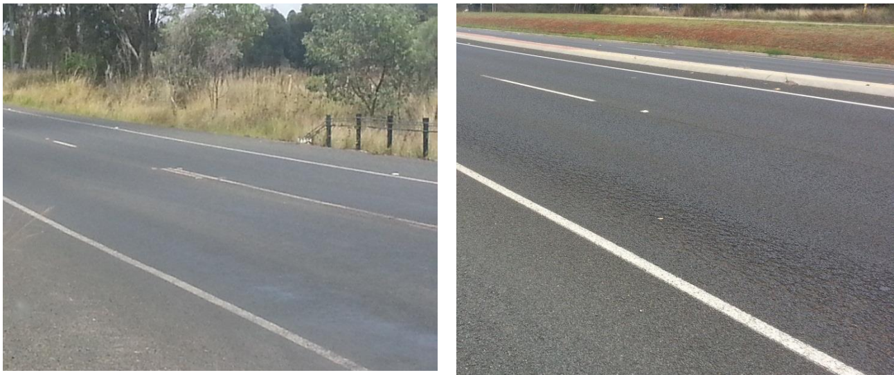
Figure C 2: Minor flushing in wheel paths and some surface deterioration in outer wheel path
